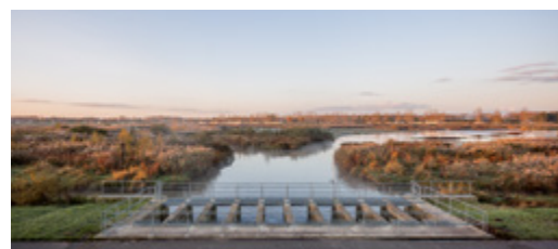
Flood area, Battel
